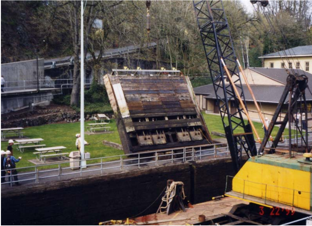
Left: Photo #4 shows the leaf being lowered onto the work area.
