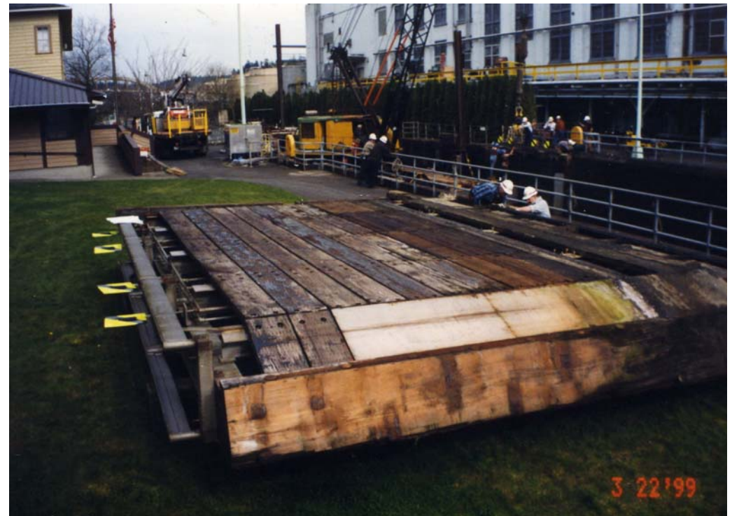
Right: Photo #5 shows the leaf being inspected.
