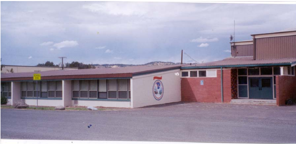
Newly painted Elementary Wing
